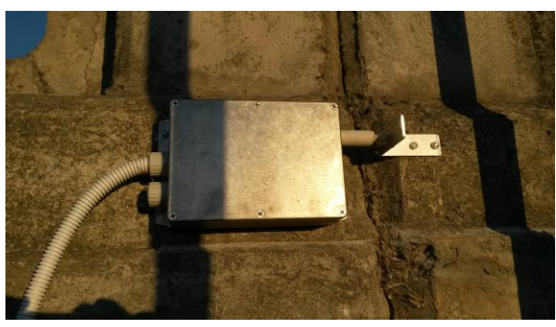
Figure 4: Permanent displacement transducer installed to monitor beam/column joint opening
