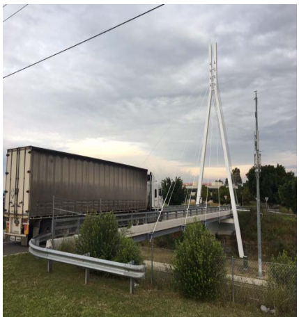
Figure 4. Proof testing using a heavy truck
