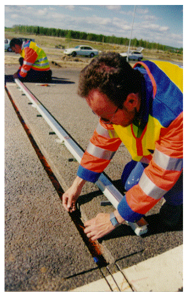
Figure 3: Installation of a pavement WIM system sensor.
