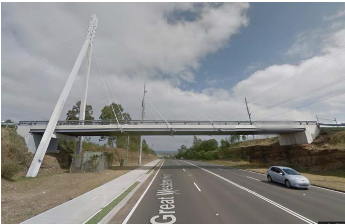
Figure 1. The cable stayed bridge at the intersection of Second Avenue and the Great Western Highway Werrington NSW (Image from Google Earth)
