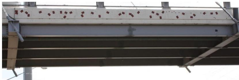
(c) I-shape steel beams and girders beneath the bridge.
