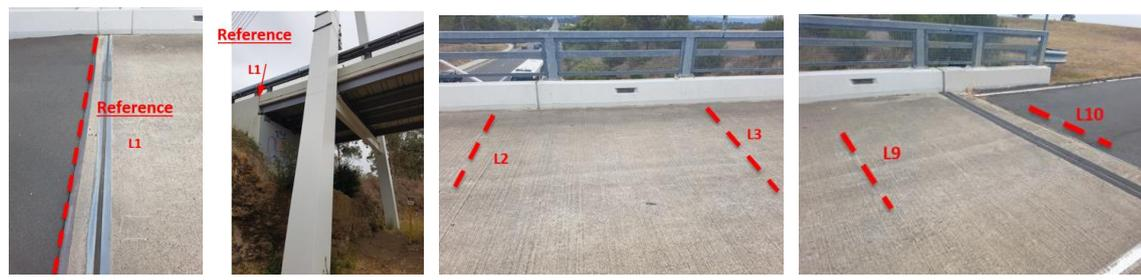
**Fig 4.** Marked lines on the bridge for loading locations.
