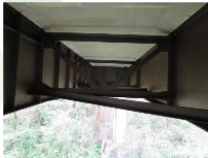
Centre of the girder
