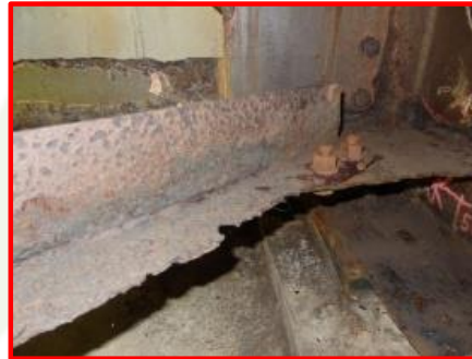
End of the girder
