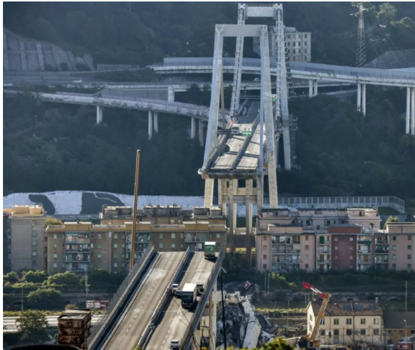
The Morandi bridge tragedy killed 43 and left 600 homeless – but also dealt a hammer blow to Italy’s engineering legacy. The Guardian . (2018)
