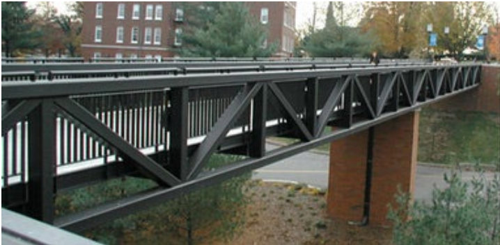
Fig.3 Overview of the Dowling Hall footbridge
