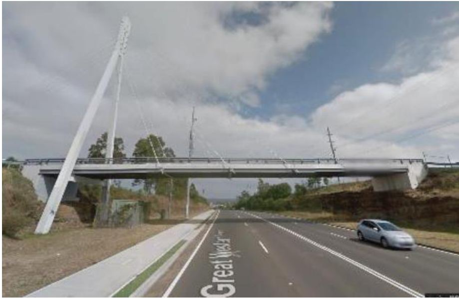
a cable-stayed bridge
