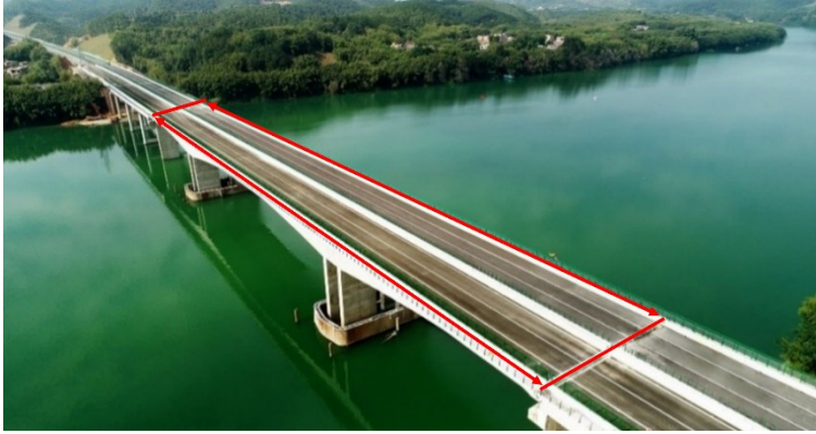
Figure 1: View of the continuous rigid frame bridge (Red box mark)
