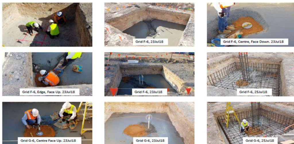
Figure 3. Installation of vibrating wire earth pressure cells underneath building footings
