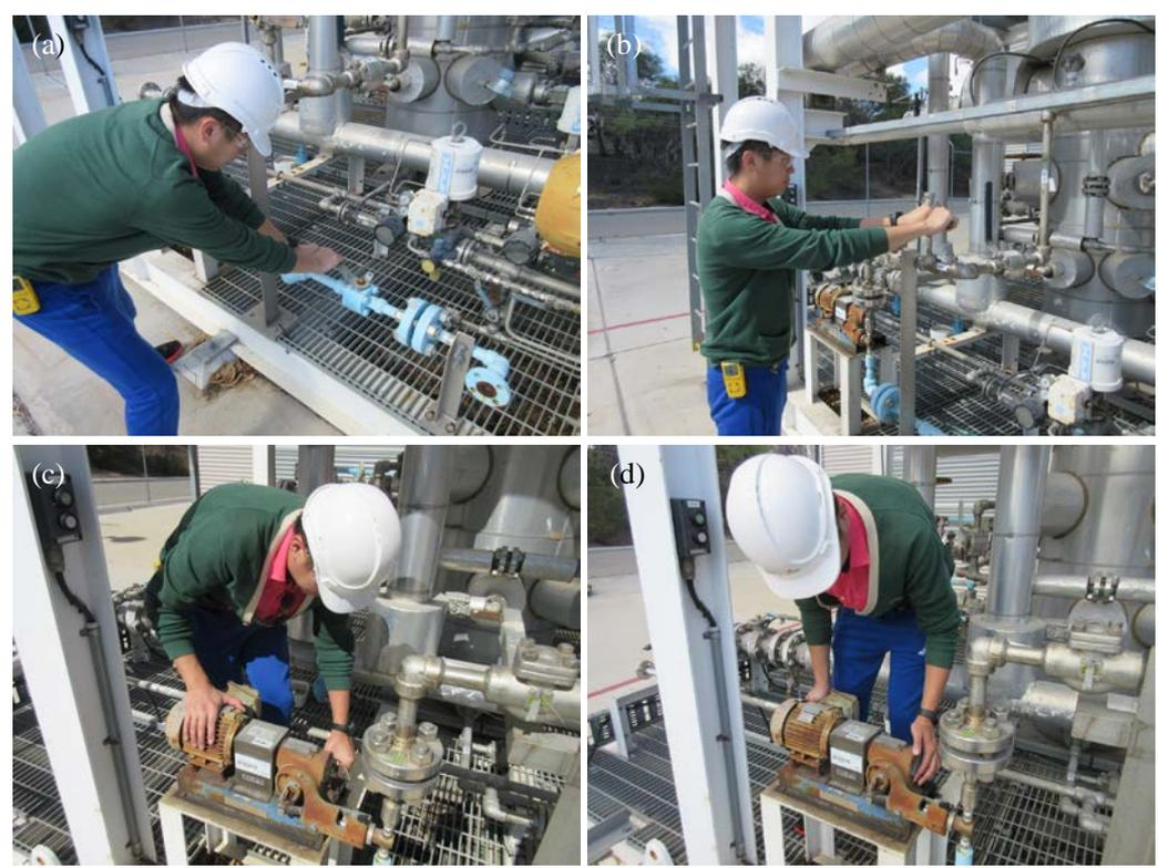
Figure 3. Simulated pump P-141 blocked-out and removal training procedure: (a) switch off the ball valve 13 and (b) 12; (c) unbolt connections of the pump and related flanges, and (d) the pump removal
