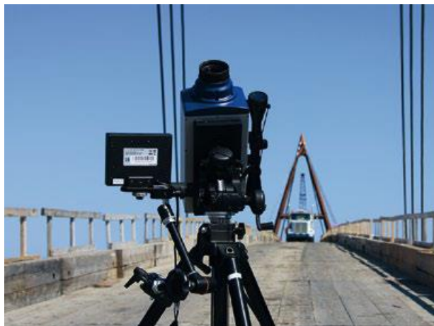
Figure 1: RSV-150 in action during the construction of the Deh Cho Bridge in Canada.
